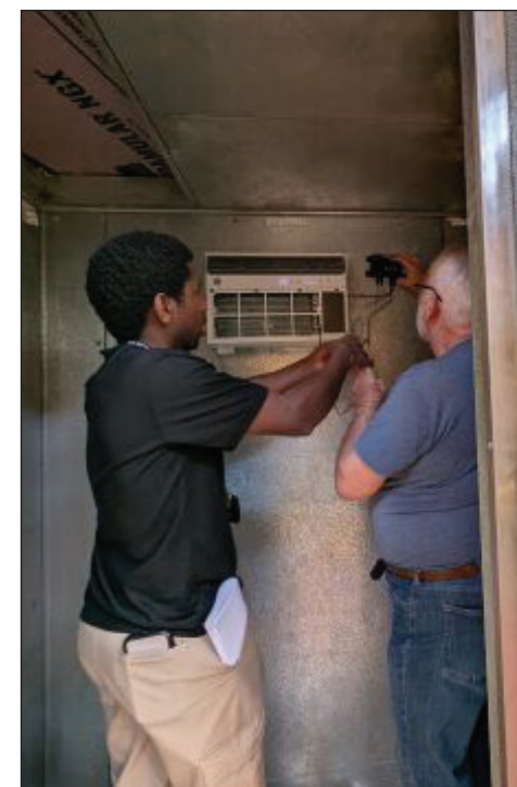
Participants installed the CoolBot to the AC unit.
